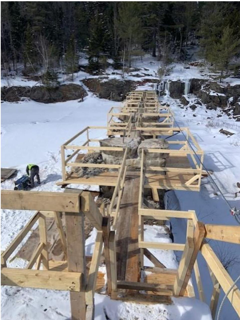
Preparation of work platforms for drilling and grouting of spillway piers - February 20, 2024
