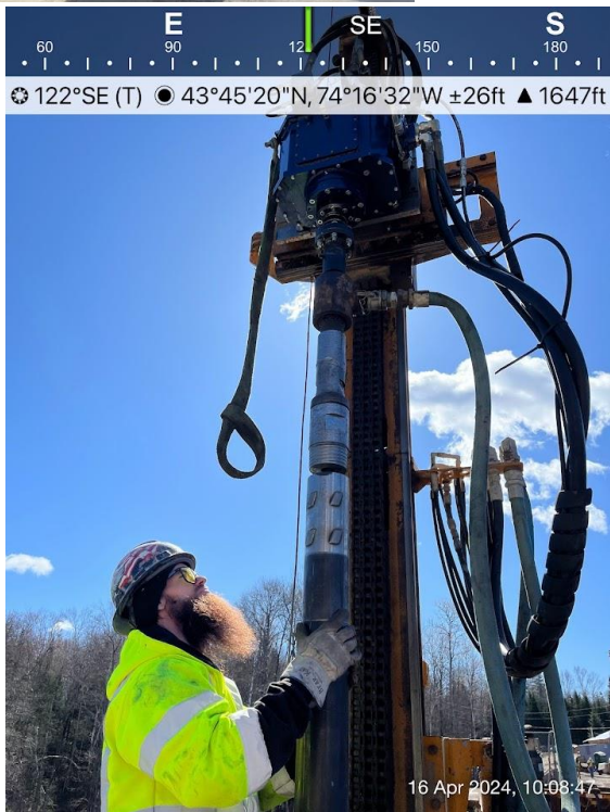
Apr 18, 2024 at 3:04:25 PM 198 Indian Lake Dam Rd Indian Lake NY 12842 United States Pressure Grouting @ P-7 5-10
