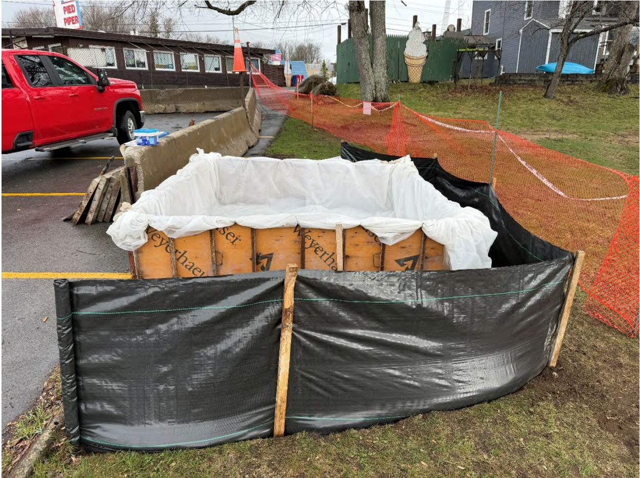
Completed sediment basin.
