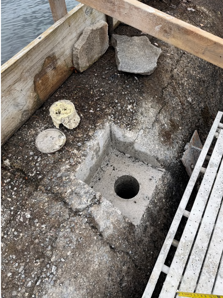
Completed anchor pocket at south location.
