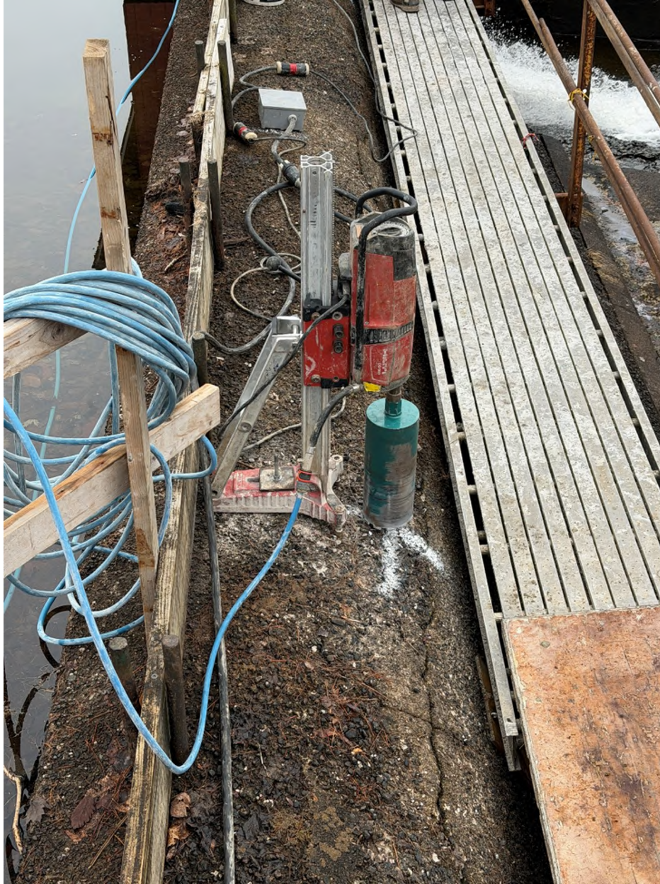
Coring setup at north location.
