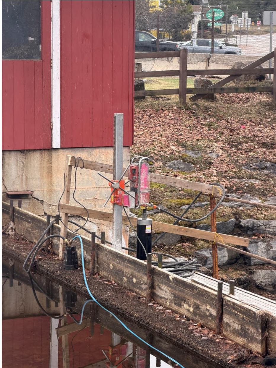
Coring setup at south anchor location.
