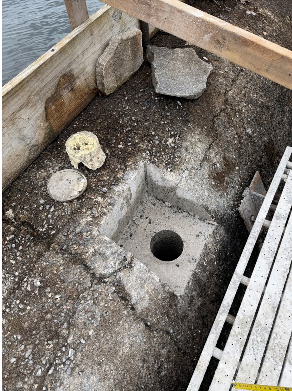
Completed anchor pocket at south location.
