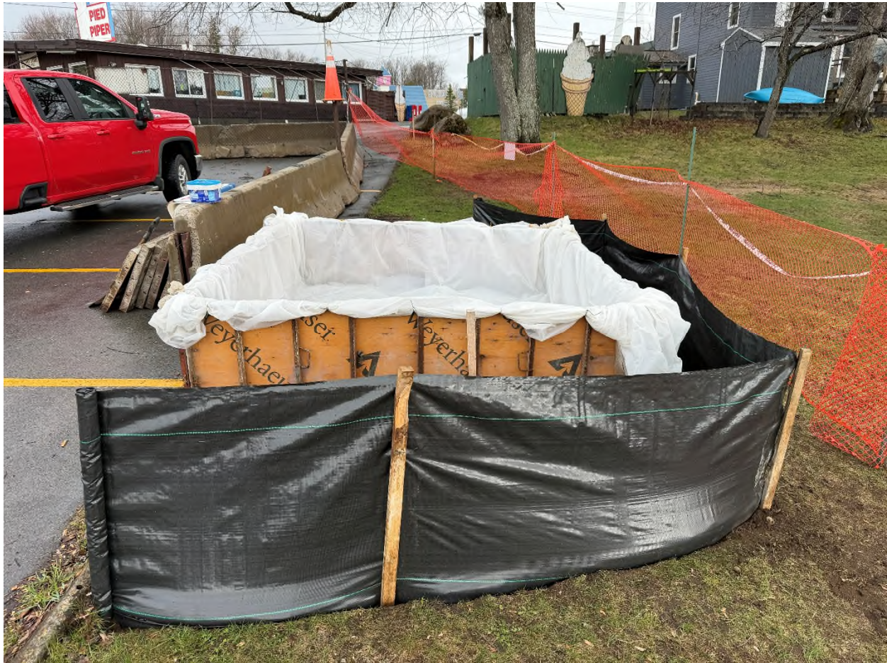
Completed sediment basin.
