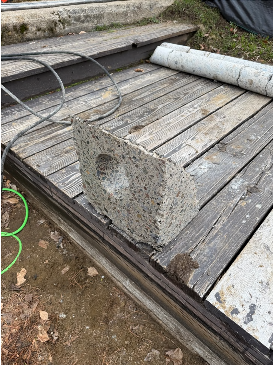
Concrete removed from anchor pocket.
