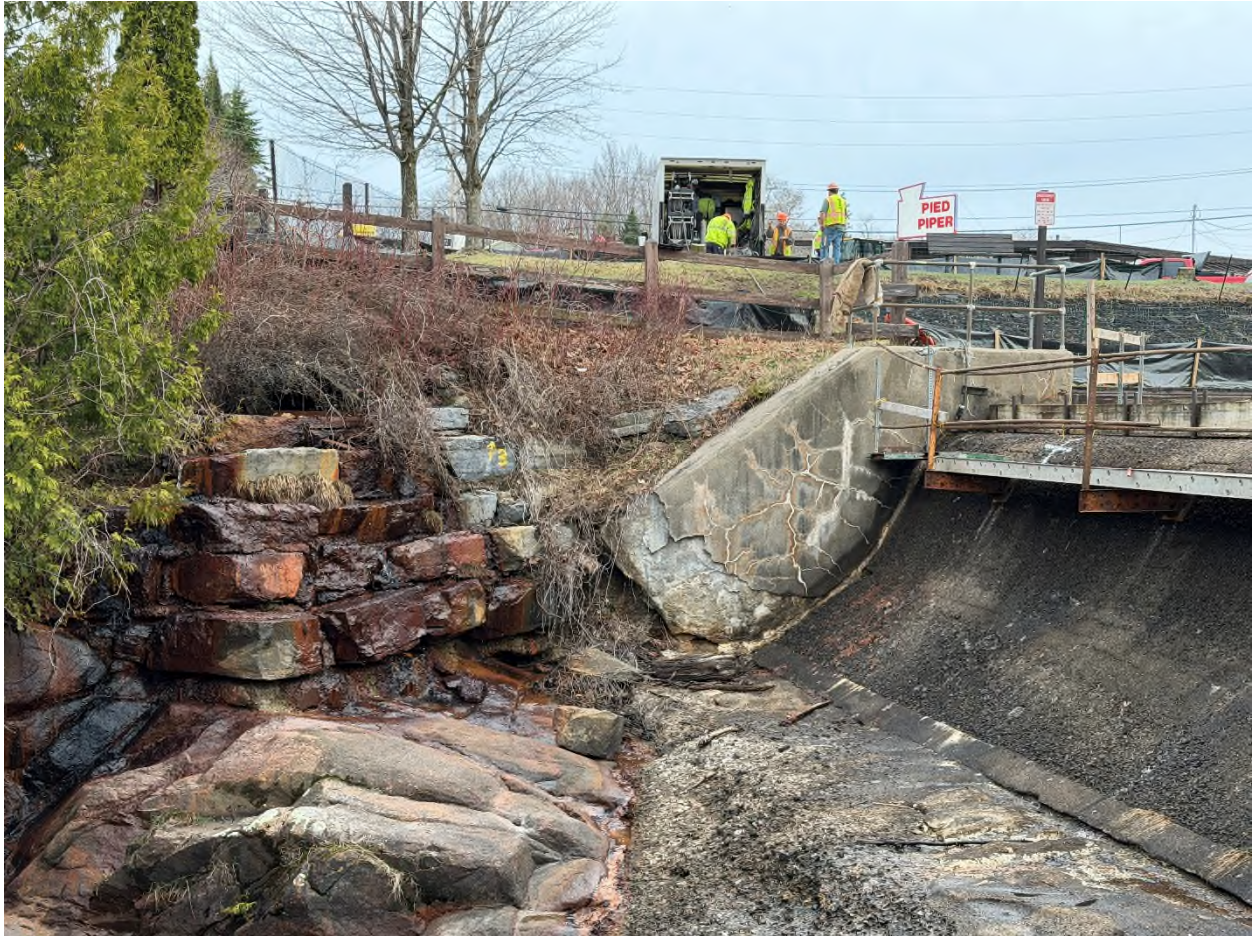
Old Forge Dam (downstream side) before coring setup.
