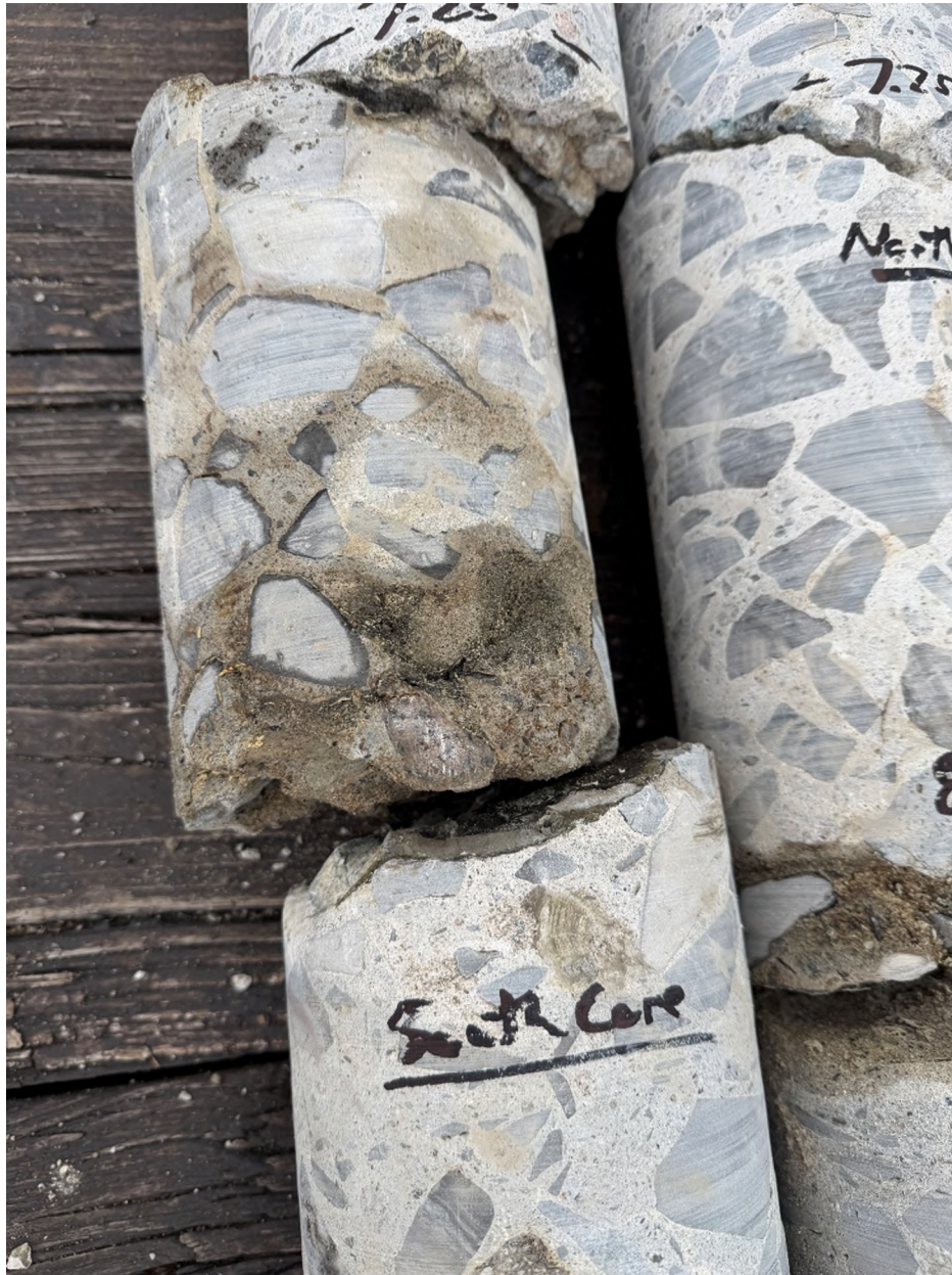
South core joint at 7.9 ft
