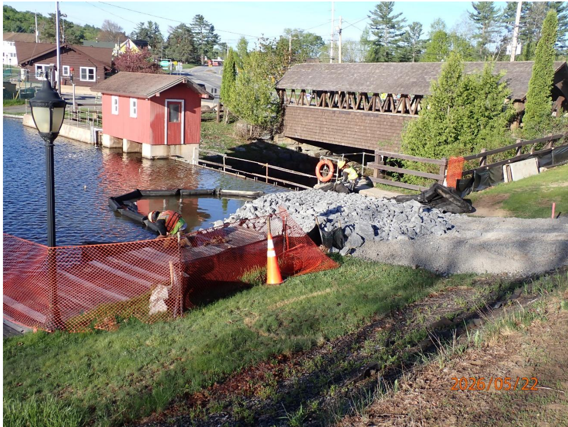
Turbidity curtain pulled into shore
