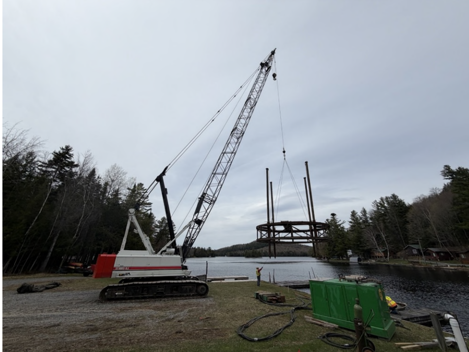
Driving template placed in lake and surveyed
