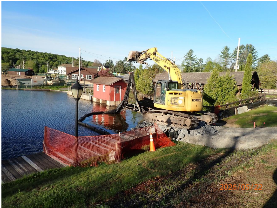
Crew pulling the turbidity curtain into shore
